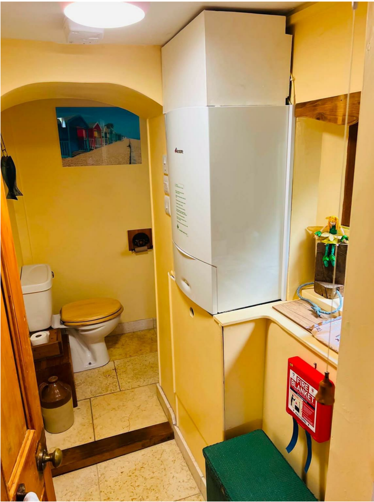
UTILITY AREA/SHOWER ROOM
