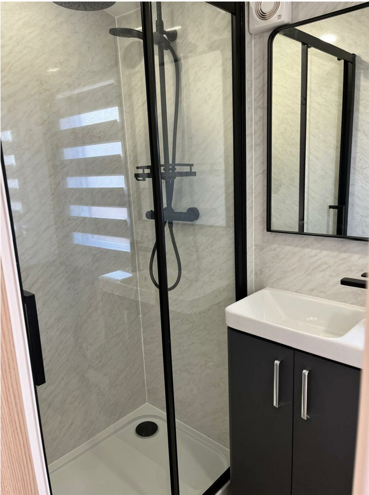
REFITTED SHOWER ROOM
