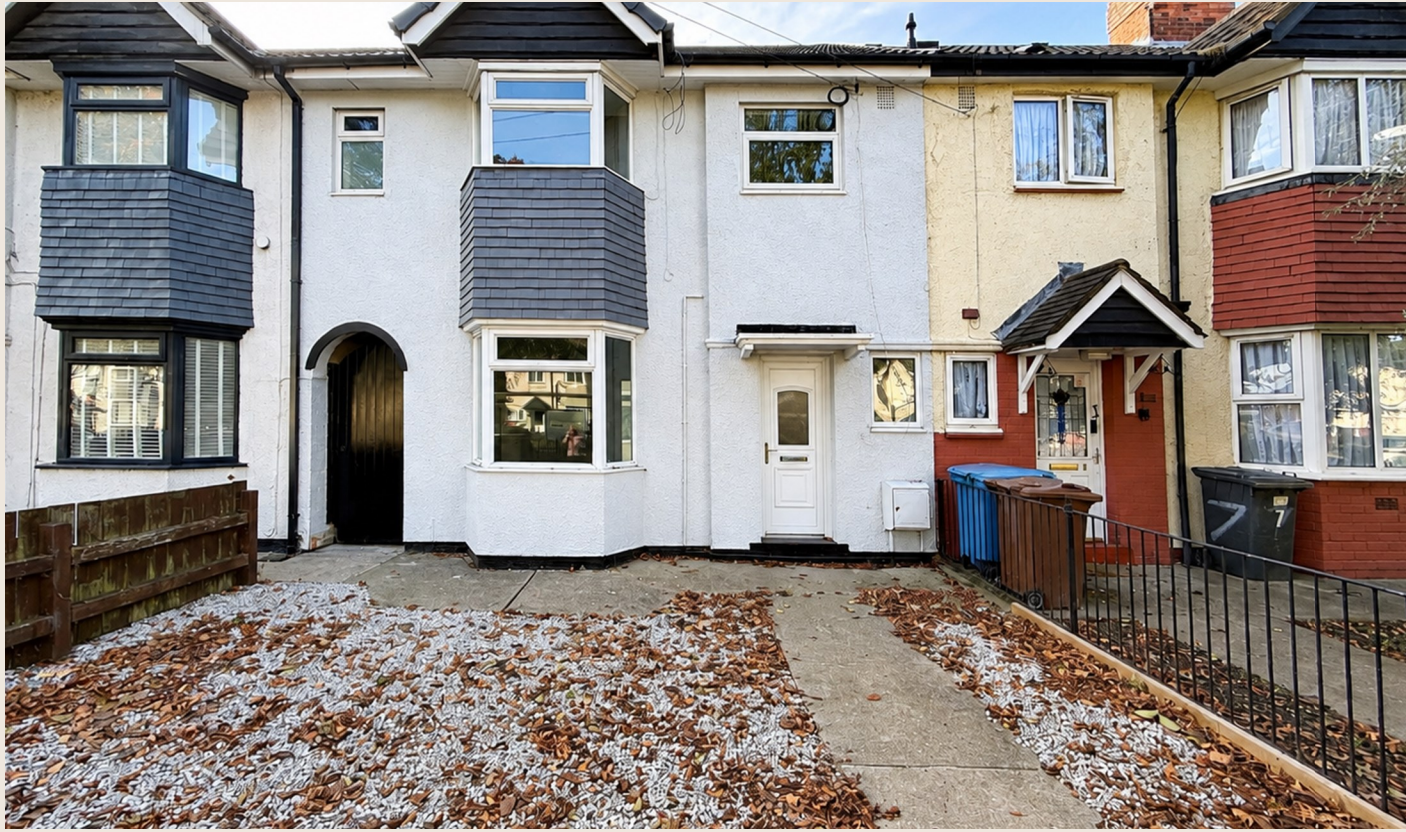
Calvert Road Hull, HU5 5DF
